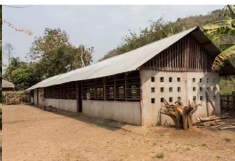
Renovated kitchen Noh Bo 2015
